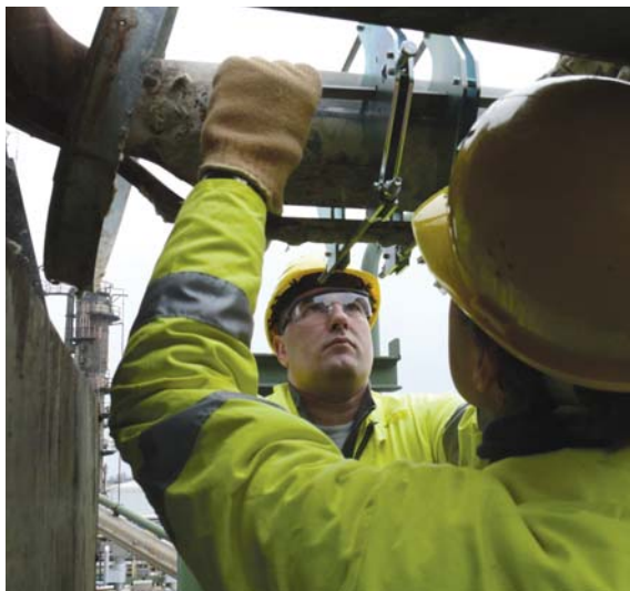
WaveInjector® and ultrasonic transducers are installed without interrupting the process
